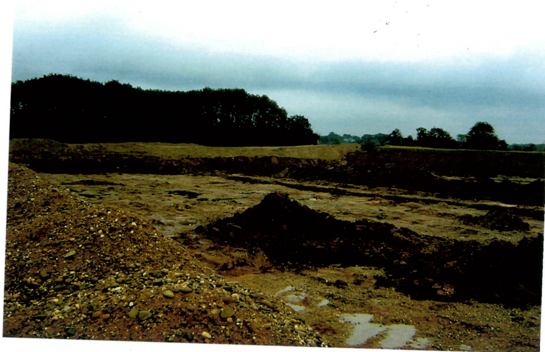
Above: A general view of the workings, September 2003.
